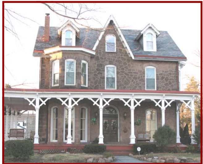
Illustration for appropriate maintenance of Historic roofing, cornices, chimney, trim and paint color. Radcliffe Street, Bristol Borough, Pennsylvania
