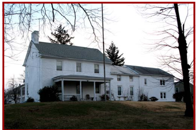
Stucco Finish: Farmhouse , West Circle Bristol Borough, Pennsylvania.
