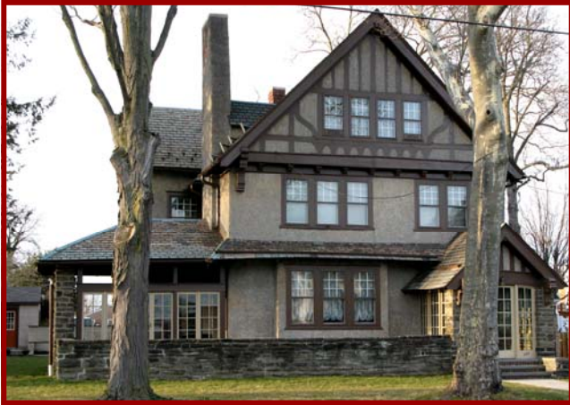
Tudor Revival, Radcliffe Street, Bristol Borough, Pennsylvania.
