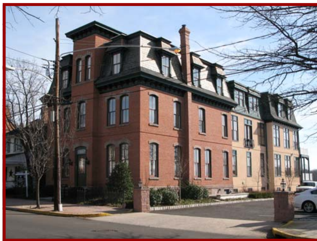
Illustration for Building Height and Form - Addition: An addition to a historic building should be a secondary form that preserves the form of the historic building. A
