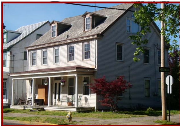
Wood siding, metal roofing, original window trim, porch and posts. Dorrance and Cedar Street Bristol Borough, Pennsylvania.
