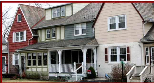
Harriman Historic District, Row homes along Wilson Avenue. Wood siding, stucco, ornamental half-timbering and slate roofing.
