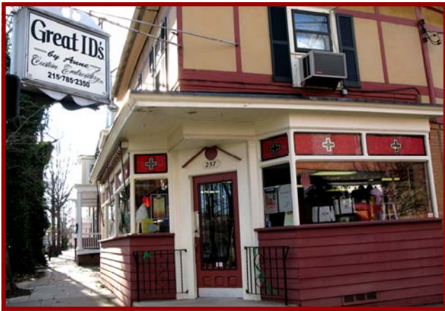
At left : Radcliffe & Mulberry Street, Bristol , PA Gift shop with appropriate maintenance of stucco, paint , drainage and preservation of original use of the shop.
