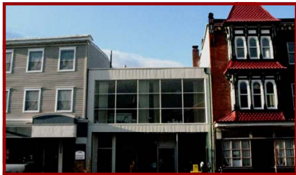
Illustration for Visual Relationship between “Old & New” The inappropriate massing, size, and storefront configuration of the new building is incompatible with neighboring structures and diminishes the historic character of the block. This is a perfect example of a 20th Century Commercial property that now has historic relevance.
