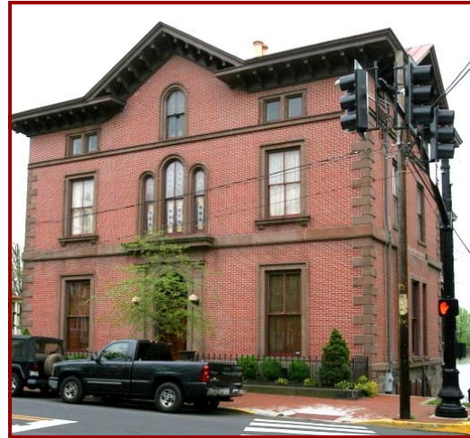
The Dorrance Mansion, 300 Radcliffe Street was entered onto the National Register of Historic Places in 1986.
