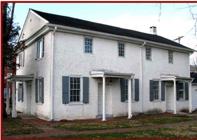
Friend's Meetinghouse, Bristol, Borough, Pennsylvania. Built 1711. Proper installation of gutters and down- spouts.
