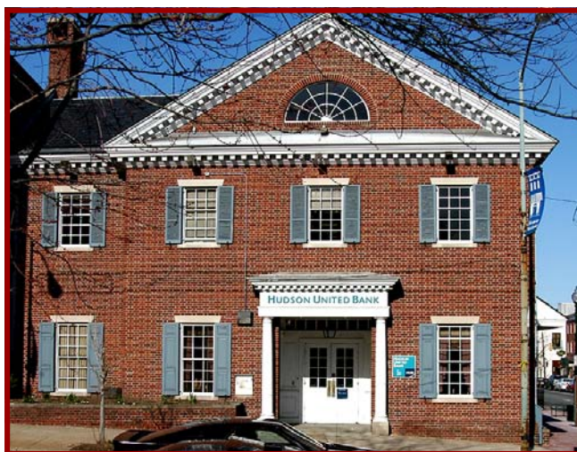
Illustration for Replicating Historic Buildings: Though not a replica of a historic structure, this new building exhibits a false historical character. This approach to contemporary design is not encouraged. Image courtesy of Design Guidelines Writer.
