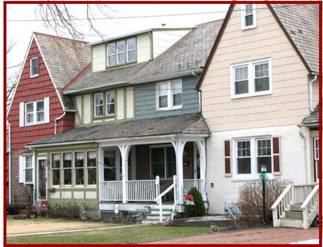
Illustration for Roofs-Dormers: The overall width of a proposed shed dormer should not exceed one-half of the roof width.
