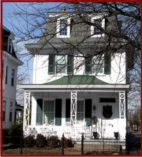
Windows and Shutters: Proper configuration of multiple panes and custom sizing. Shutters are correctly sized, appear workable and appropriate materials used.
